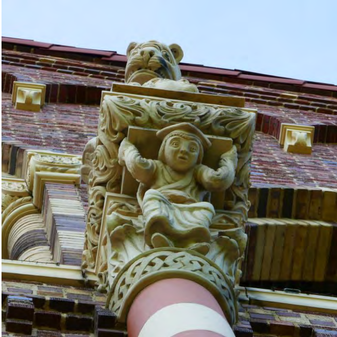
Figure 9. "Final Exams," west façade. Source: Corbett AHS, Inc.
