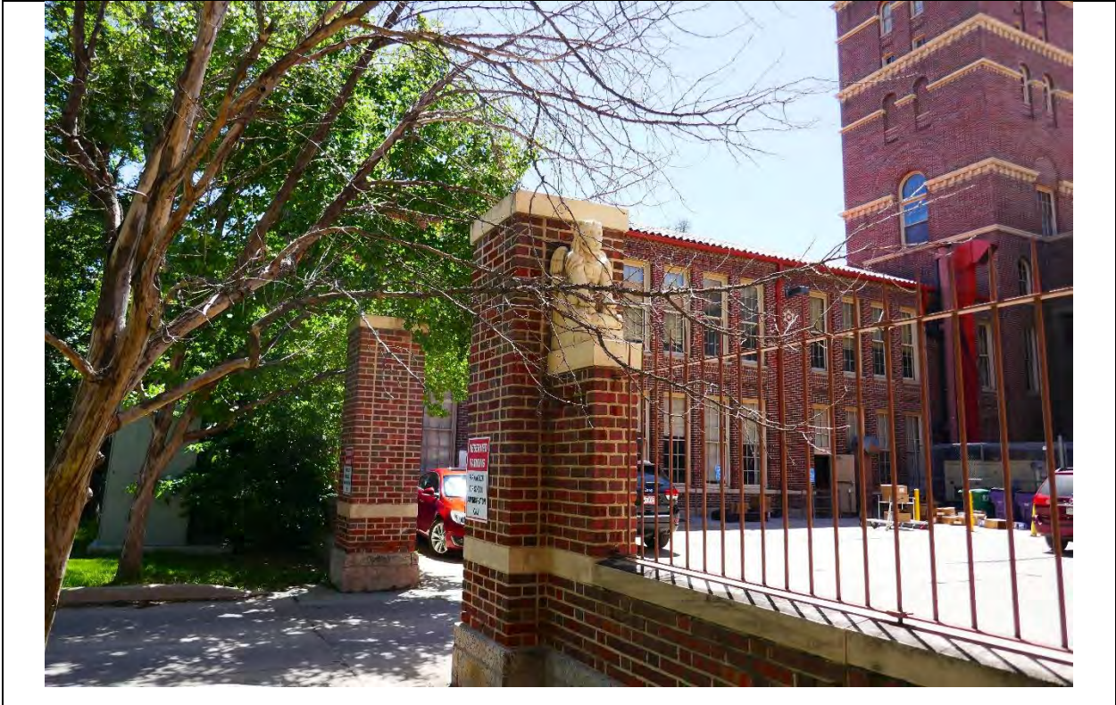
16 6/16/2022 Facing ESE Detail: Gargoyle at north parking lot fence
