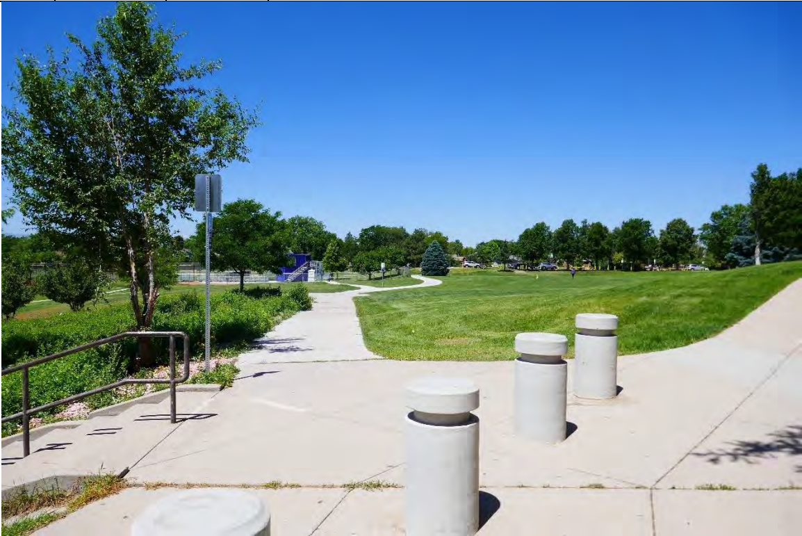
57 6/16/2022 Facing W Walkway along the south of the resource boundary
