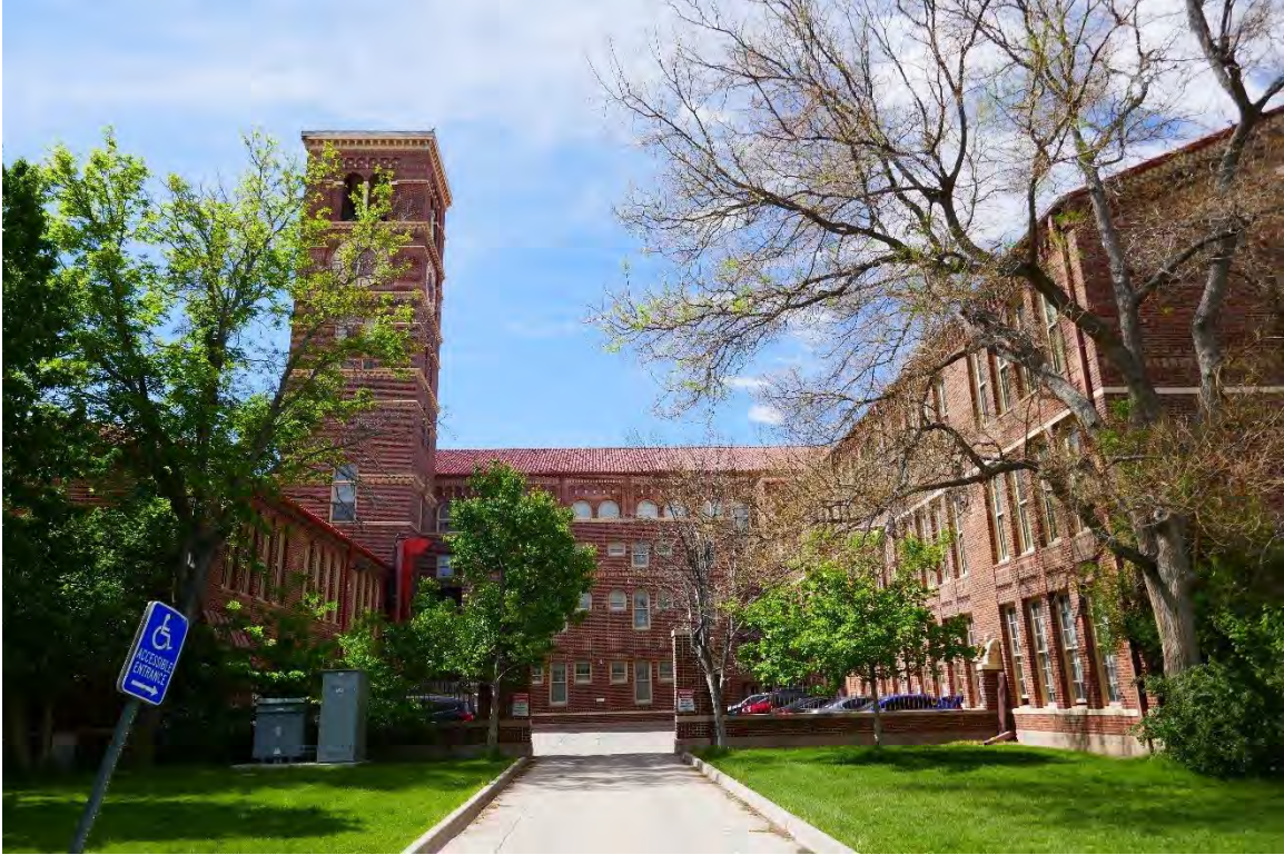
14 5/27/2022 Facing S North courtyard/parking lot; north façade between wings
