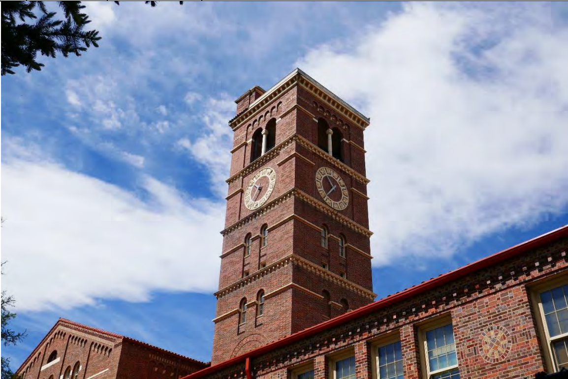
19 5/27/2022 Facing SW Clock tower, east and north sides
