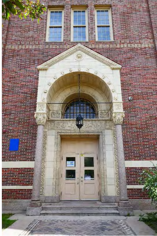
12 5/27/2022 Facing S Northwest entrance
