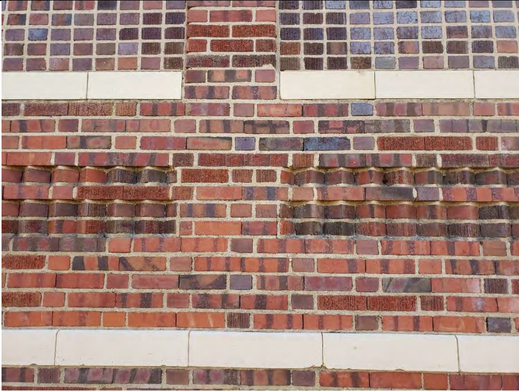
2 11/10/2020 Facing E Detail of brickwork, west facade
