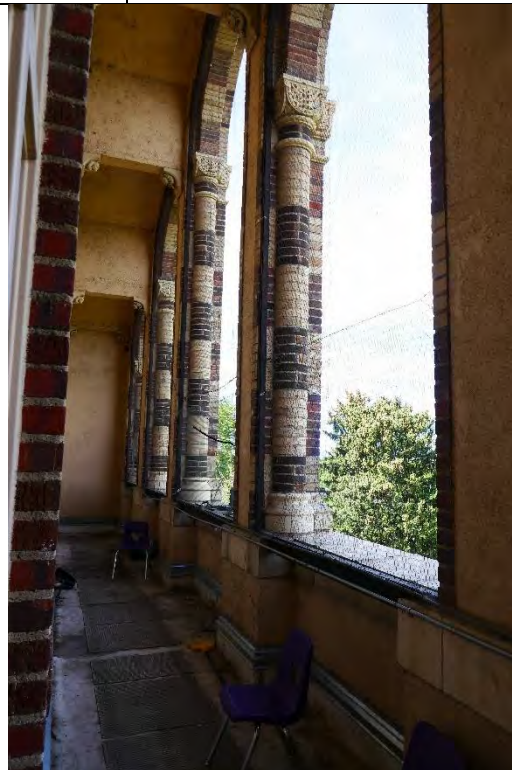
37 5/27/2022 Facing SSW Inside the loggia above the main entrance
