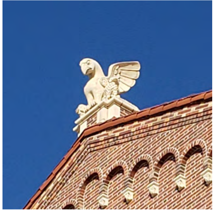
Figure 10. "Gertie Gargoyle" on the roof peak, west façade. Source: Corbett AHS, Inc.
