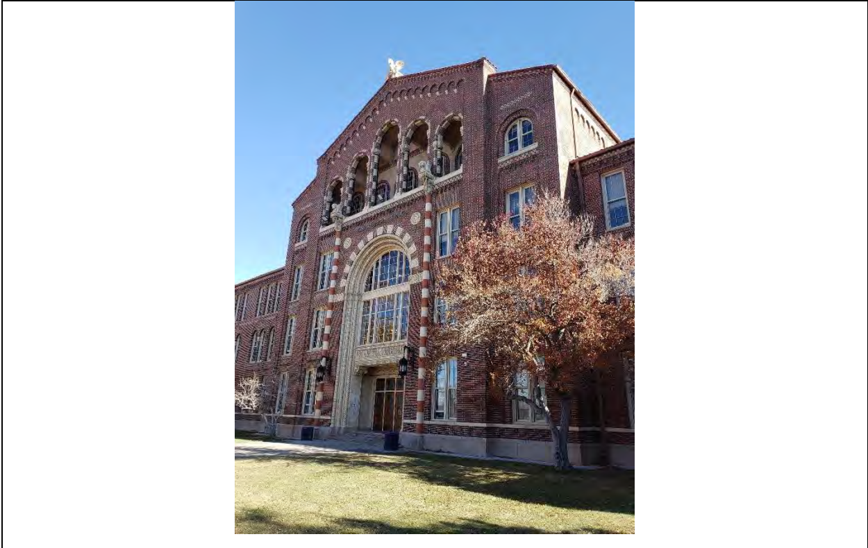
4 11/10/2021 Facing NE Primary façade and main entrance
