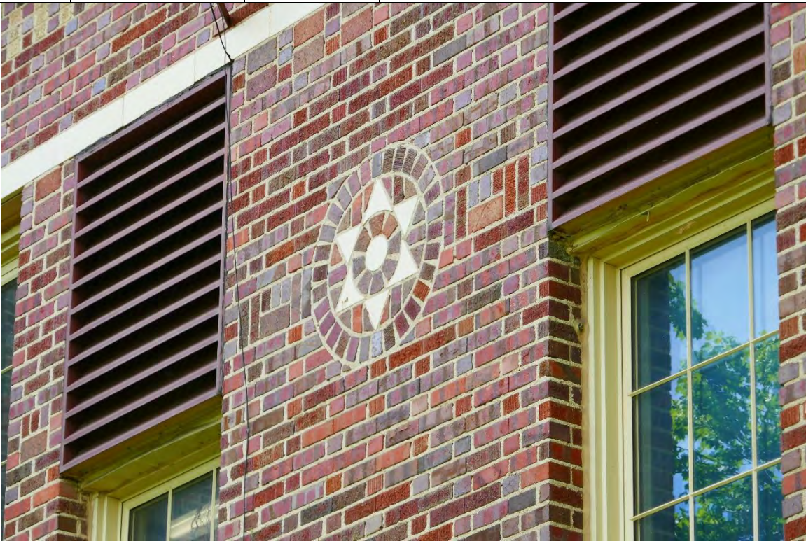
3 5/27/2022 Facing ENE Detail of brickwork, Star of David, north facade
