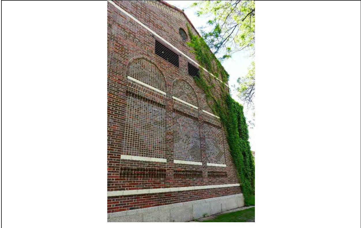
8 5/27/2022 Facing SSE Detail, West Façade, west side of north el
