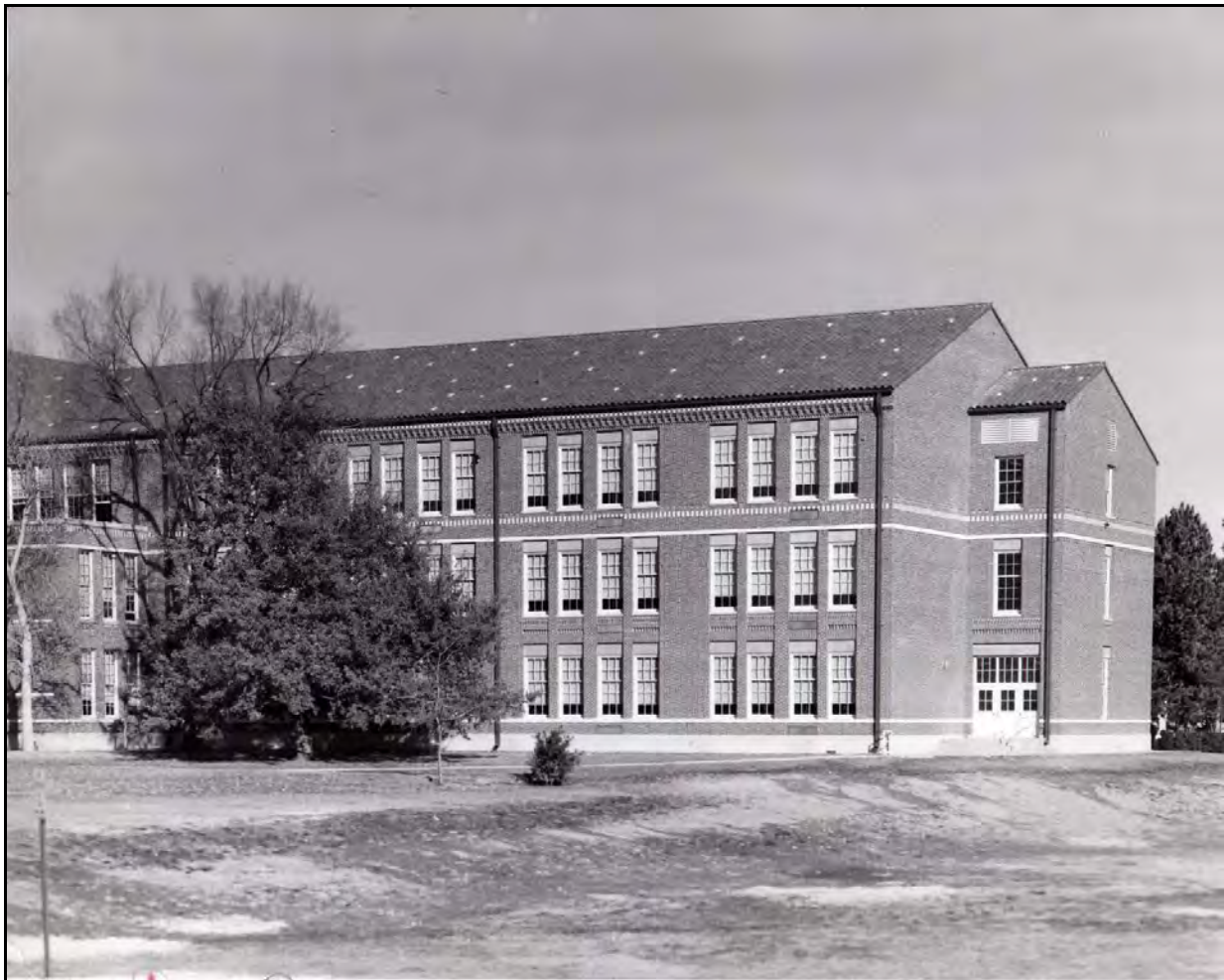
Figure 15. South addition to the high school, designed by Charles Gordon Lee and completed in 1963. Source: SHAFI collections.
