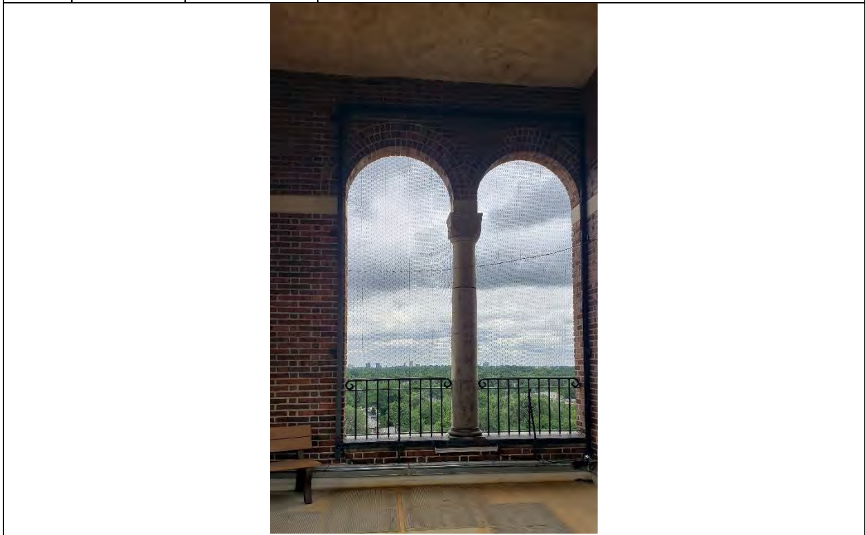
21 6/21/2021 Facing E The view east from the top story of the clock tower
