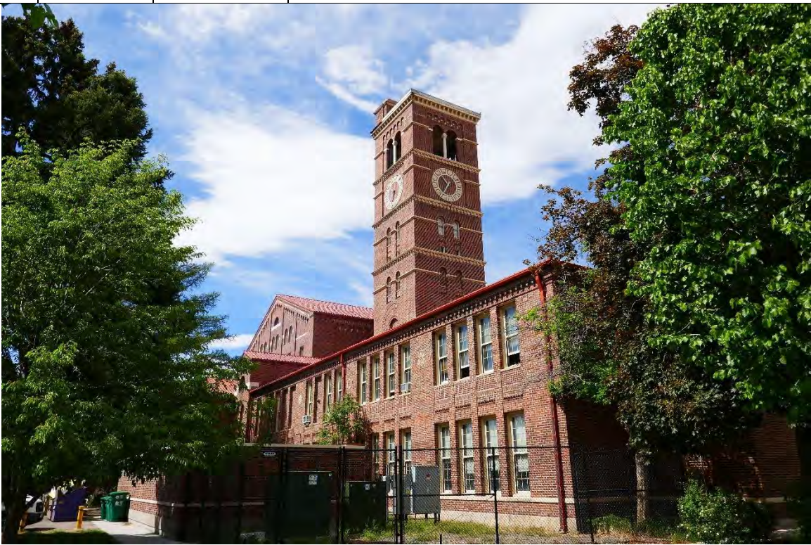
23 5/27/2022 Facing SSW East façade, north wing showing clocktower
