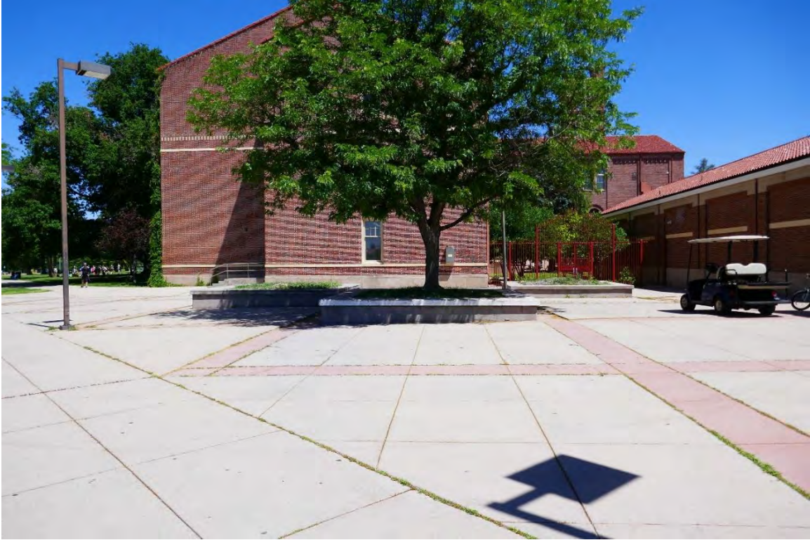
60 6/16/2022 Facing N Triangular landing area at the south end of the 1963 classroom addition, showing the three raised planters (noncontributing)
